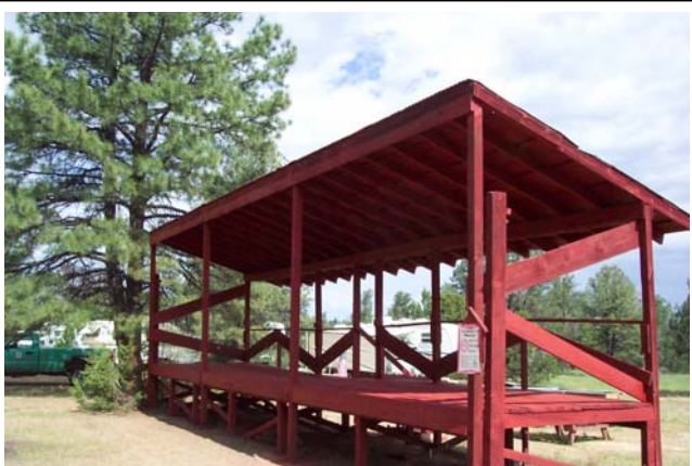
Covered stage, improvements: roof, stairs, and paint.
