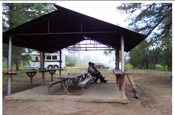
Ramada improvements: removal of large concrete BBQ trough, replaced with picnic tables.
